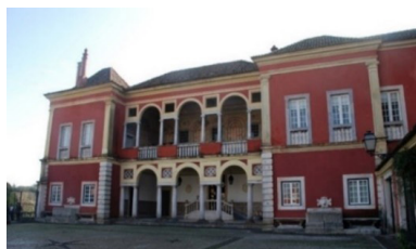
a. North Loggia façade – main entrance.
